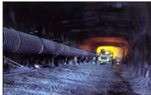
Twin two lane tunnels between Bexley Road and Marsh Street, Arncliffe
