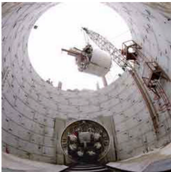
Figure 3: The Tunnel Boring Machine in the shaft at Elstree. Weighing 80 tonnes, the TBM advanced at approximately 150 m per week.
